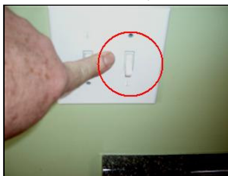
2.0 Picture 12 Broken Switch
