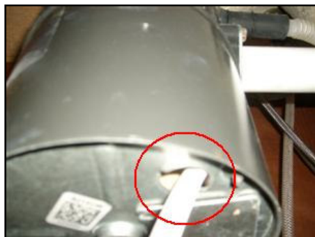
2.0 Picture 7 Bottom of Disposal
